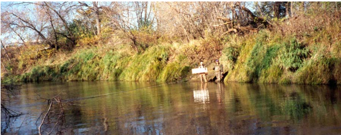
Figure 6-5: Aquatic habitat sampling in reach B3 located downstream of Kindred. Note the vegetated banks stabilizing the channel. The outlet would result in increased stages of about 1 foot. Prolonged inundation would result in loss of vegetation, increased bank erosion, and sloughing
